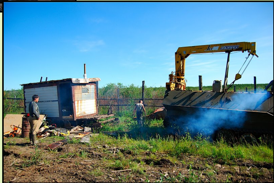
Dragging the Fish Box to the Tower Site
